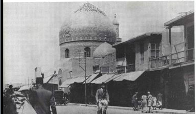
A SCENE IN BAGHDAD. Carter's have recently shipped to Dhibban, near this ancient city, the materials for three standard Squash courts.
